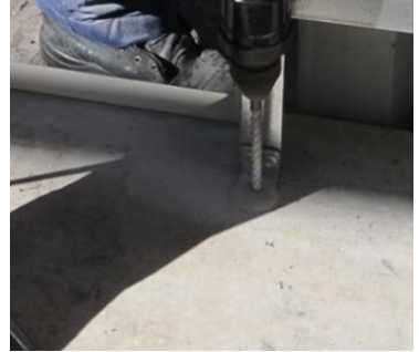
12. Install the dynabolts
