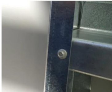
10. Tek on the holding down bracket
