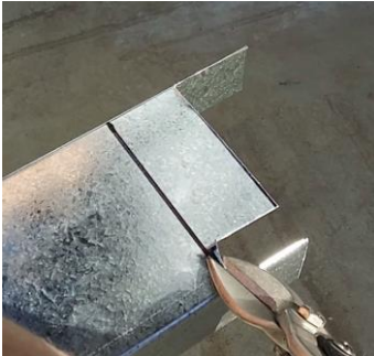
3. Install the j-flashing
