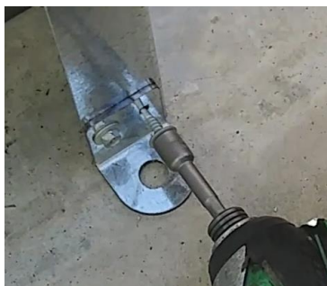
10. Tek on the holding down bracket
