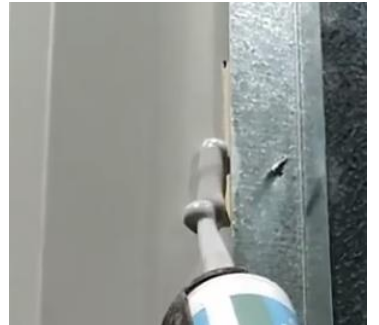
13. Silicone j-flashing (back)
