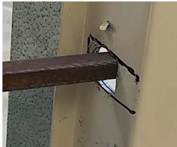
9. Tek the door jamb on to the Z's
