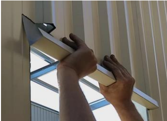
3. Install the j-flashing
