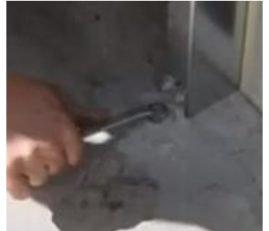
13. Silicone j-flashing (back)
